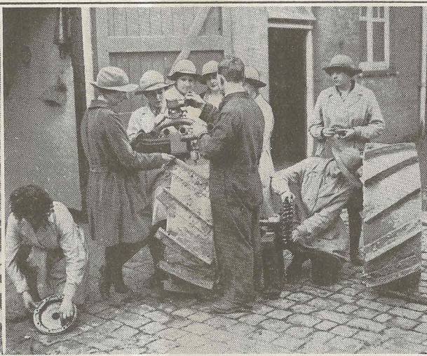
Right—Examining details of the Tractor, the Instructor explaining the operation of the Paraffin Carburettor.
